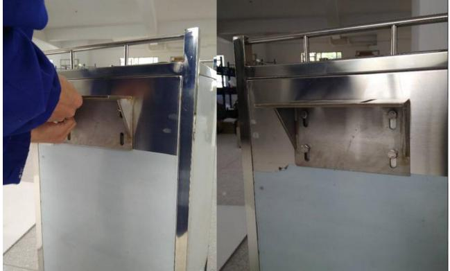
The installation of the lifting frame.
